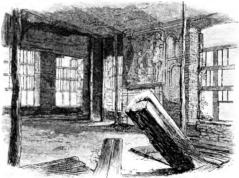
Interior of the Old Hall.
